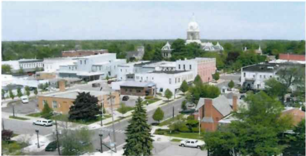
Elm St Reconstruction
