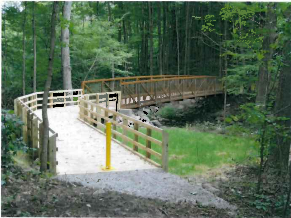
Pedestrian Bridge over Sessions Creek at the Ionia Recreation Area
