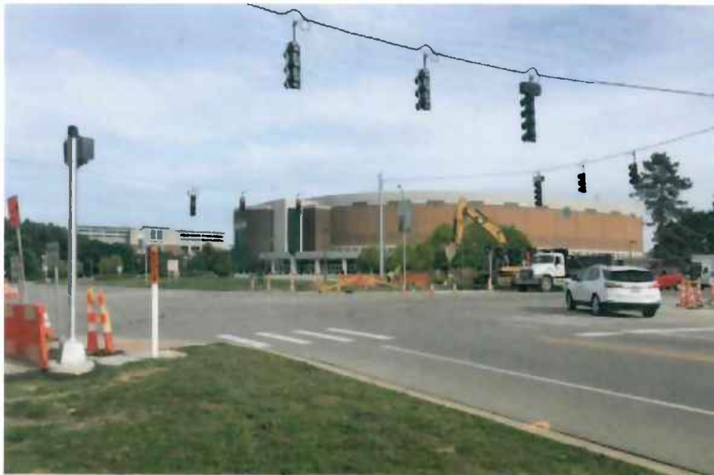
Harrison Road and Kalamazoo Street Signal Improvements
