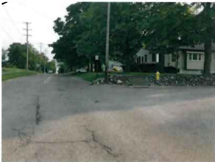
S Jefferson Street – Pre-construction, City of Mason
