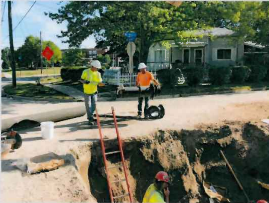
Grand Ledge Road and Utility Reconstruction
